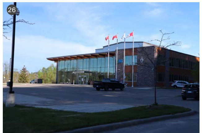
Public buildings form community focal points and should be treated with high-quality design
