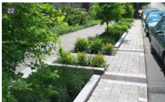
Bioswales and other measures should be incorporated to provide lot-level stormwater management control
