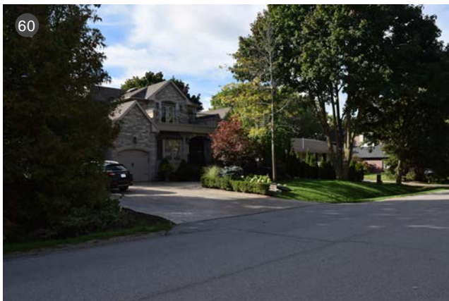
Permeable surfaces, retention of vegetation, and native plantings will promote sustainability in the Established Neighbourhoods
