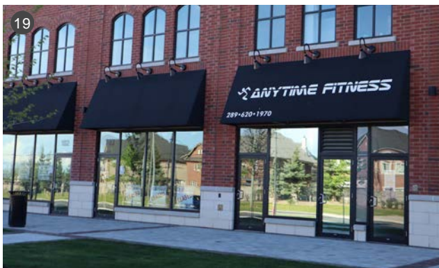
At-grade entrances, automatic door openings and hardscaping reduce physical accessibility barriers
