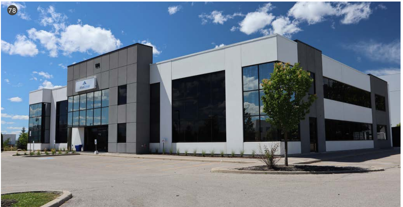
Roof pitches should be in keeping with the overall architectural design of the building
