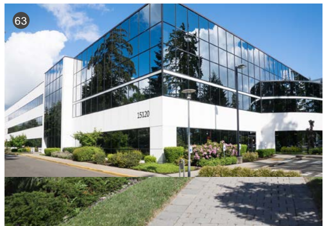
Landscaped areas provide a visual buffer and assist in stormwater management
