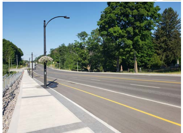
Utilities are encouraged to be buried to improve the aesthetics of the public realm. The images above contrast the aesthetic difference between overhead wires (above) versus buried wires (below).
