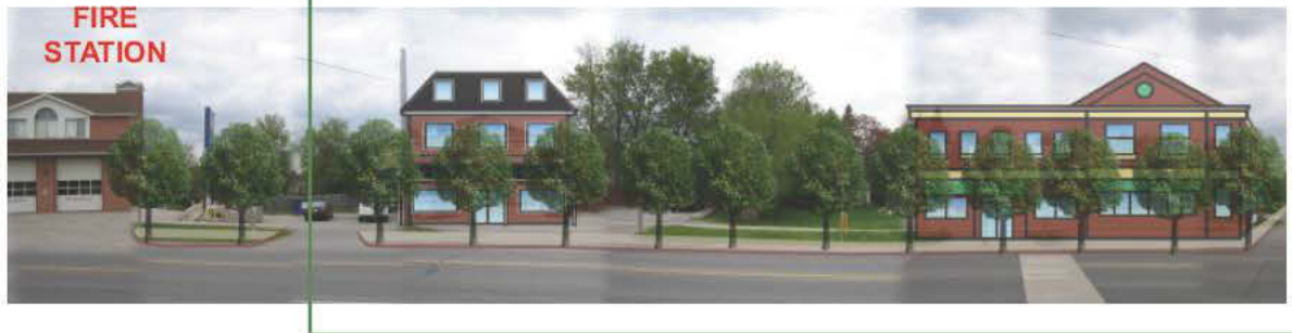
Figure 6.10 - North Side of King Road - East of Highway 27 , continued from above
