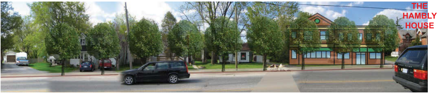
Figure 6.8 - North Side of King Road - West of Highway 27
