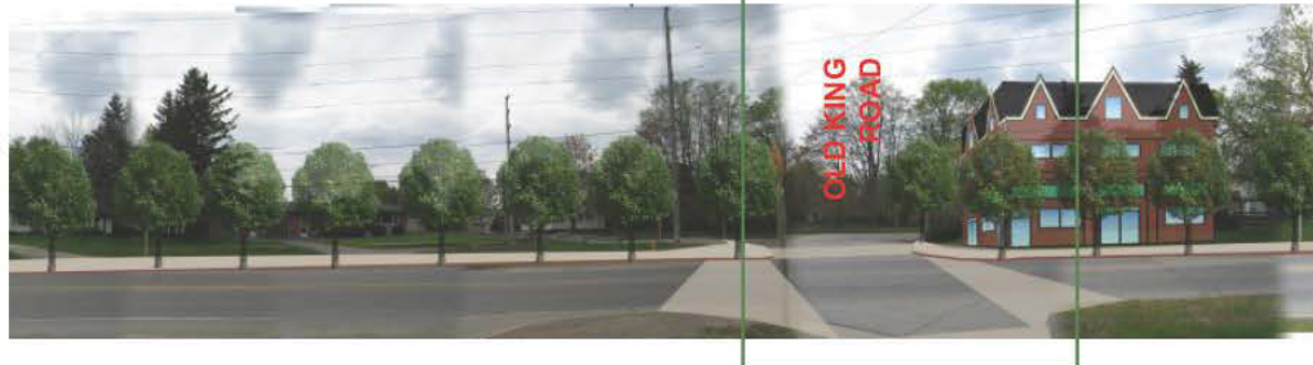
Figure 6.11 - South Side of King Road - East of Highway 27
