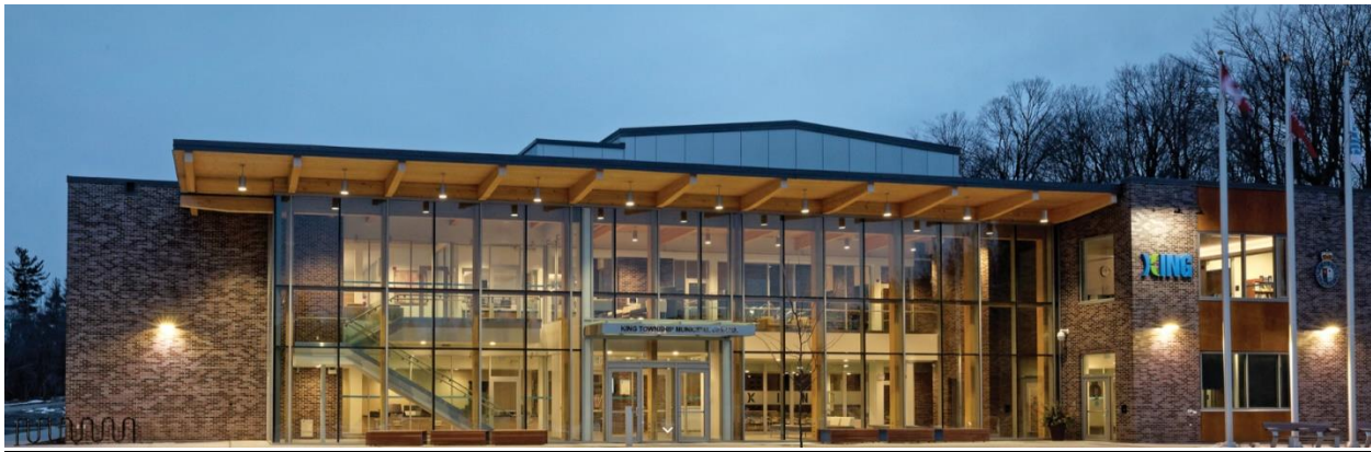
King Township Municipal Centre (KTMC)
