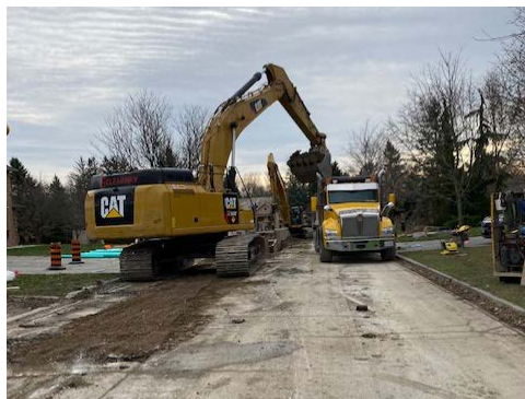
Nobleton Sewers Construction
