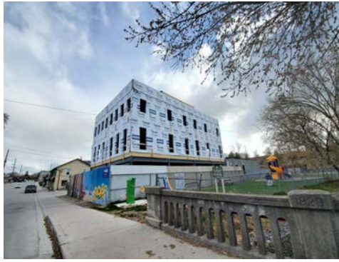
New Construction of 215 Main Street
