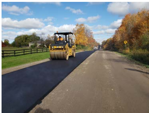
New pavement on the 11th Concession
