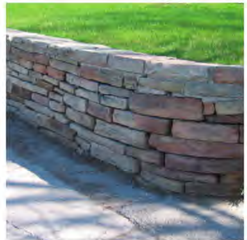
Figure 4.29 The existing stone wall on King Road is a wonderful means of transitions heights. A more durable natural stone retaining wall product should be used to maintain the look and feel of the original wall in the event it needs to be replaced.
