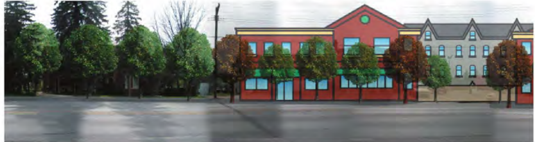
FIGURE 6.17 - WEST SIDE OF KEELE STREET ENDING AT KING ROAD
