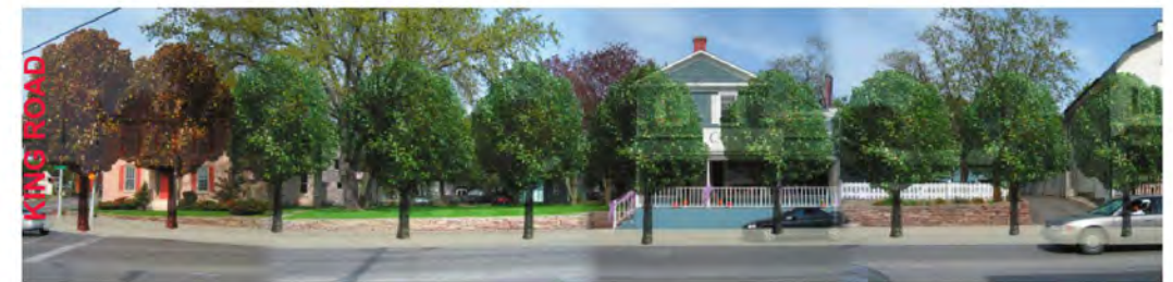
FIGURE 6.18 - EAST SIDE OF KEELE STREET ENDING AT KING ROAD
